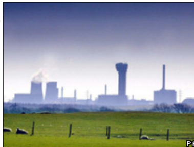
Tests were carried out between the 1960s and 1990s, said BNFL
